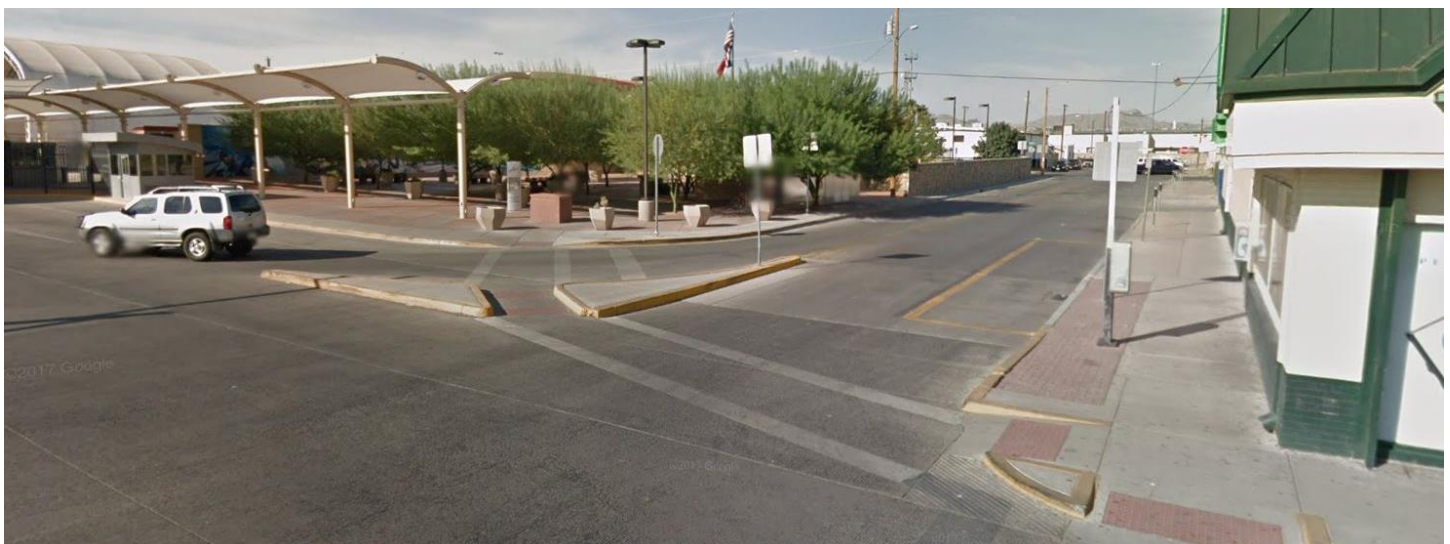
FIGURE 5.16: BIKE/PED CONDITIONS AT STANTON STREET POE ENTRY
