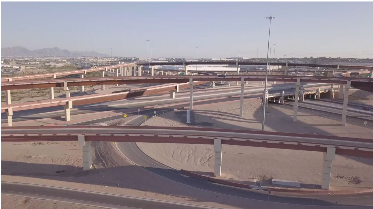
Figure 3-21. IH-10 and Loop 375 Interchange
