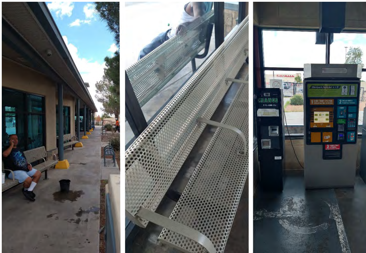
Figure 18 Arturo Tury Benavides Cielo Vista Transit Center Site Visit
