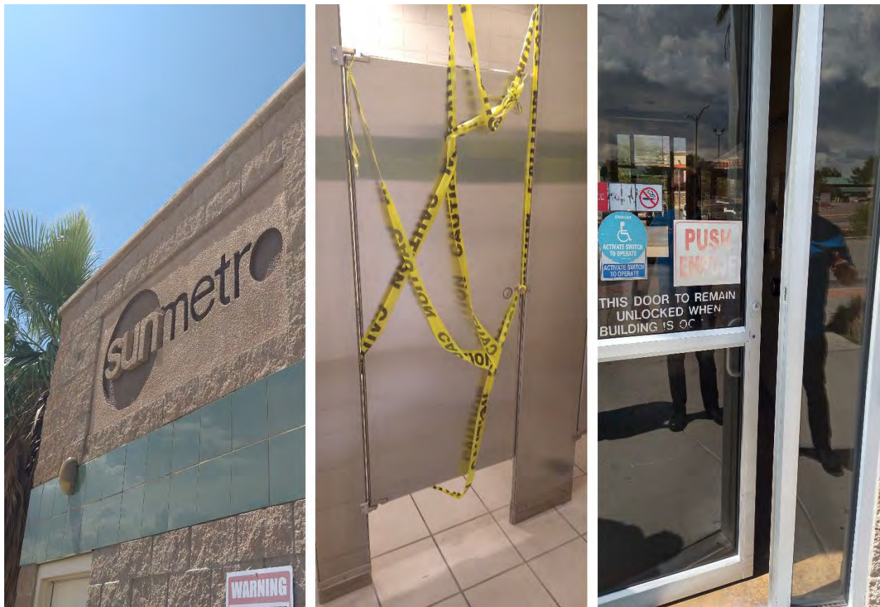
Figure 14 Al Jefferson Westside Transfer Center Site Visit
