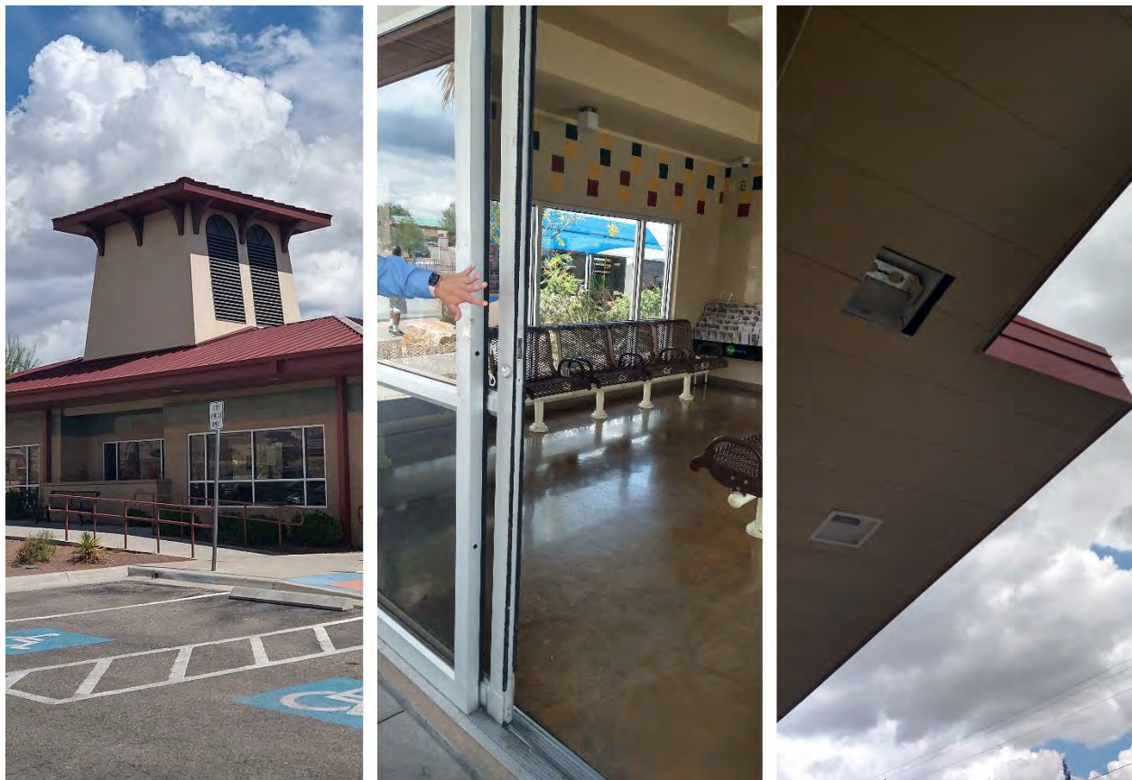
Figure 19 Robert E. McKee Five Points Transit Center Site Visit
