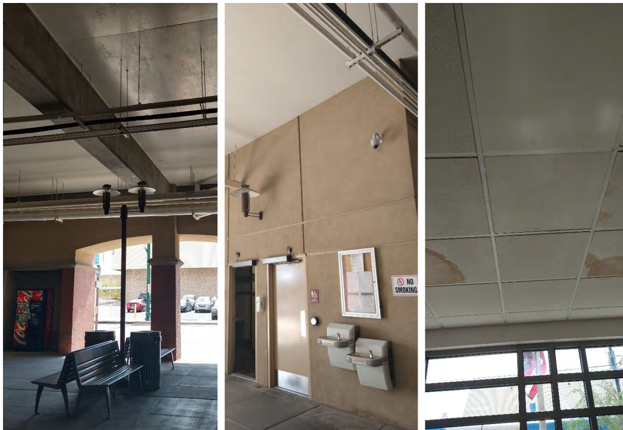
Figure 15 Glory Road Transfer Center Site Visit
